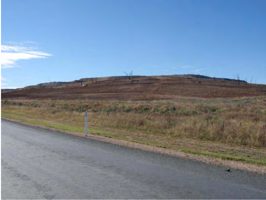
Figure 5.5 Western & Southern Rehabilitation Area after erosion repairs in May 2010
