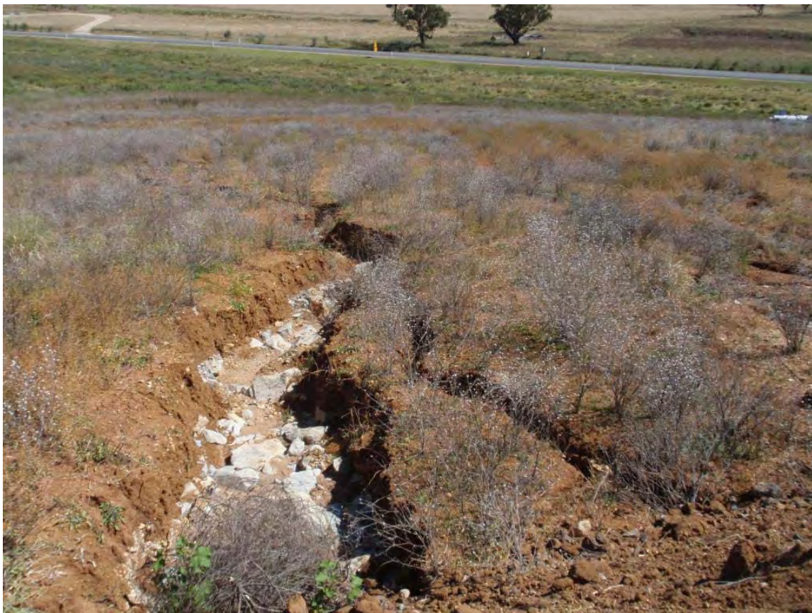
Figure 5.4 Close up of erosion and poor ground cover prior to maintenance works March 2010
