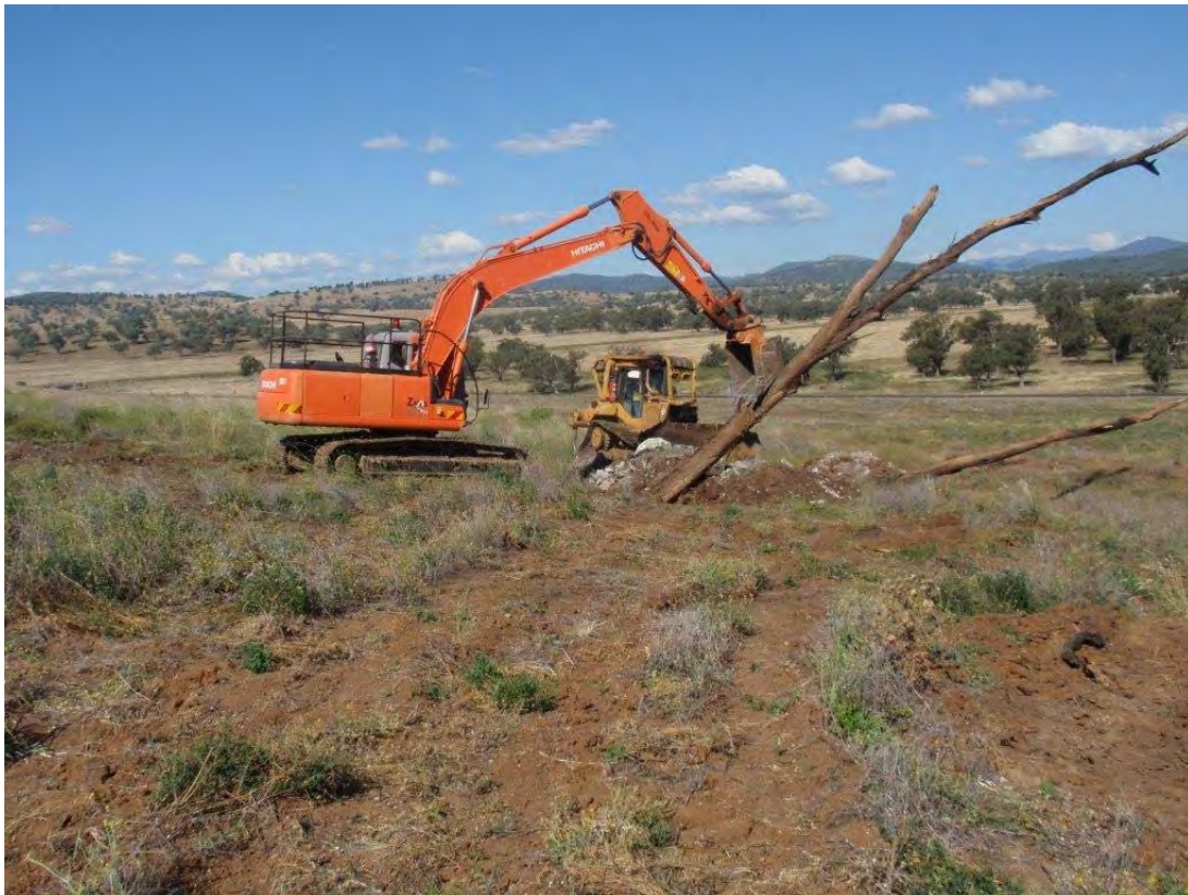
Figure 5.6 Stag Tree being installed in the rehabilitation area
