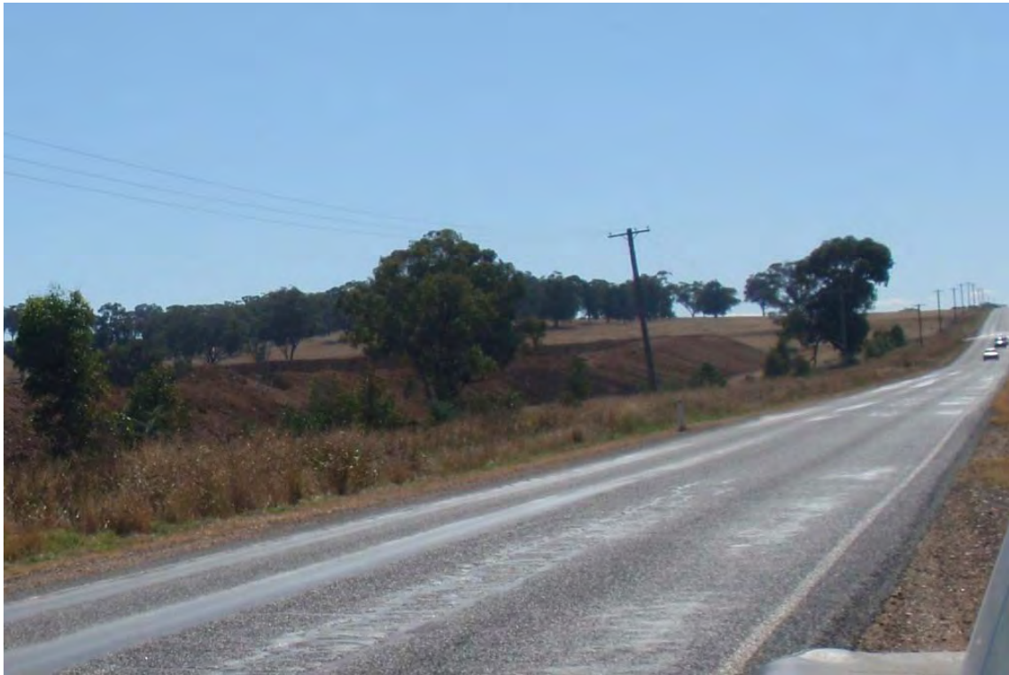
Figure 3.6 Construction of Visual Screen along Werris Creek Road at WCC
